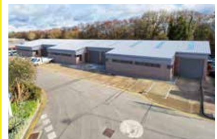
Units A-F Barwell Chessington 2338 - 14040 sq ft Fully refurbished To Let for Aviva
